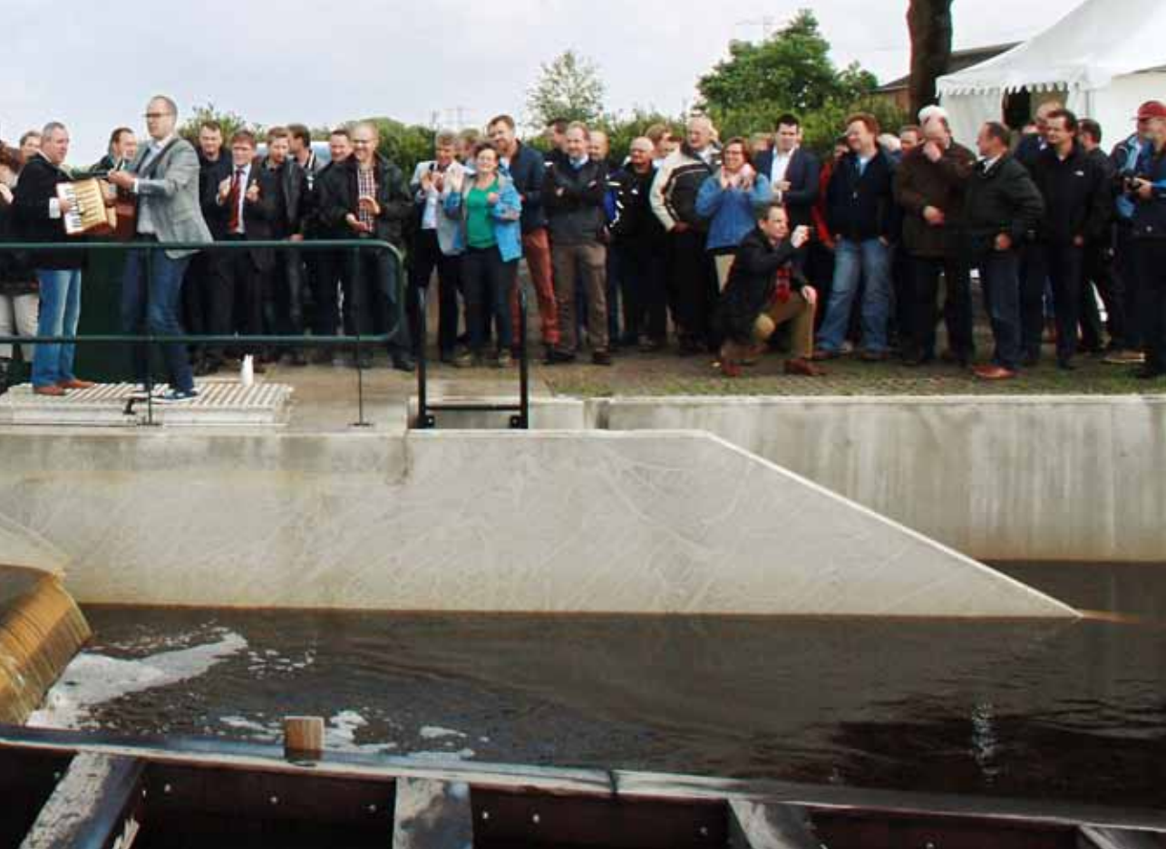
Grand opening of the project Streukelerzijl. Schoolchildren give the sign for turning on the pumpingstation
